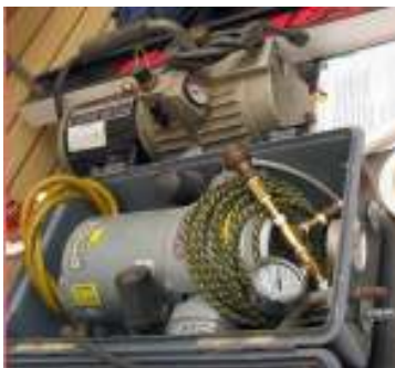
Two of three vacuum pumps demo'd
